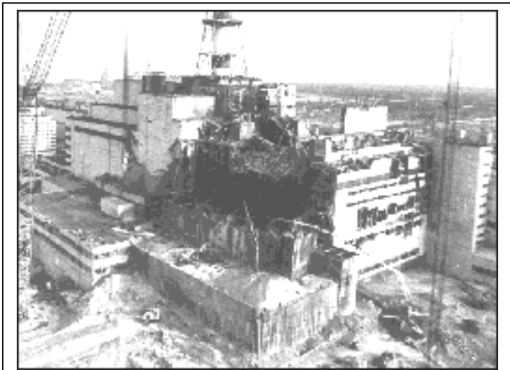
Figure 2: The number 4 reactor unit at Chernobyl. This photograph was taken when the first in the number 4 reactor had finally been suppressed. Note the streams of water directed onto the reactor from fire trucks in the hope of keeping the reactor core from re-igniting.
